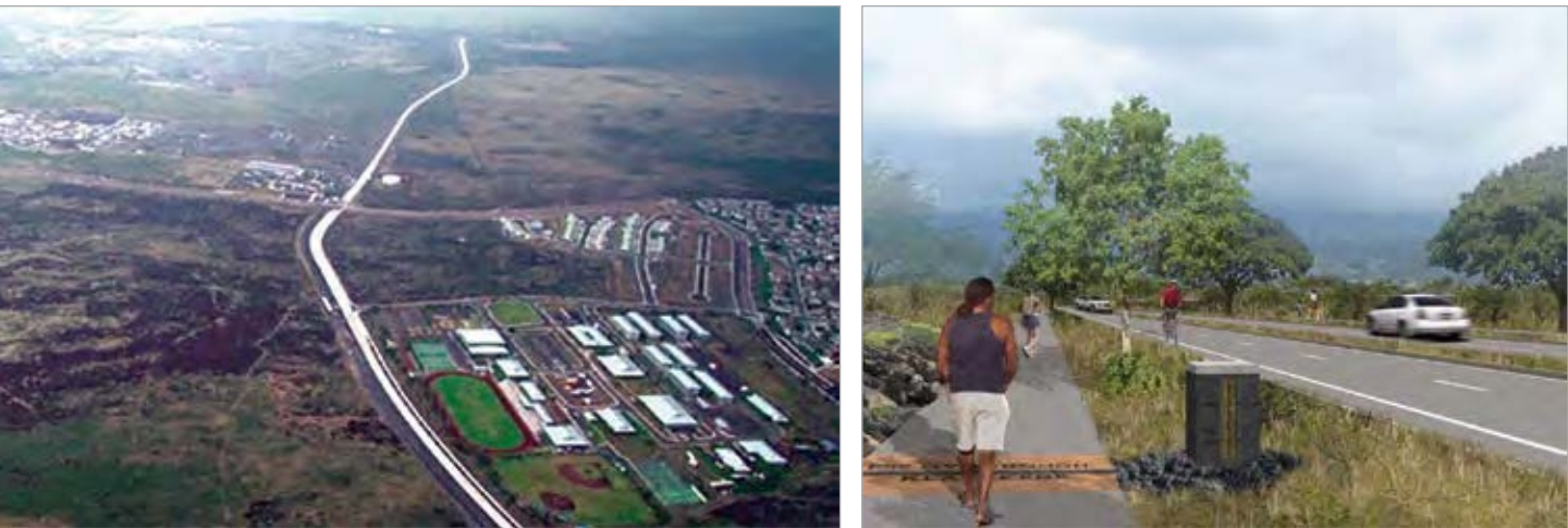
Figure 3.4-5 Ane Keohokalole Highway Corridor and Rendering of Multimodal Street Improvements, North Kona Source: Hawaii Planning Department
