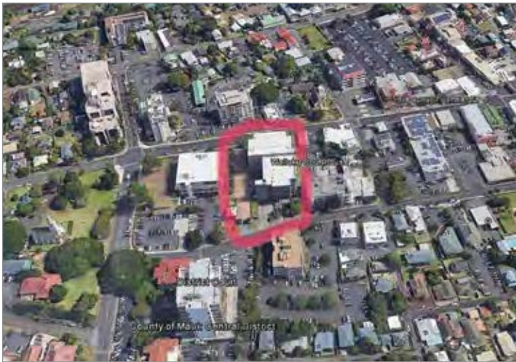
Figure 3.5-6 Wailuku Civic Center: Site of Wailuku Courthouse Expansion
